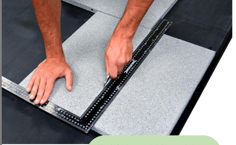
When the far edges are reached, tiles may need to be cut to suit. Use a sharp knife or for large quantities a circular saw. Ensure the bevel edges are always aligned with each other.
